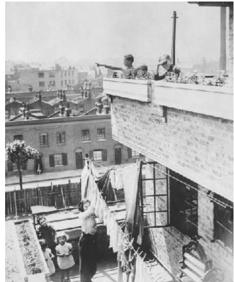
▲ Figure 1.3 View of the terraced balconies in Bethnal Green and East London Housing Association flats at Brunswick Street, Hackney, July 1936
