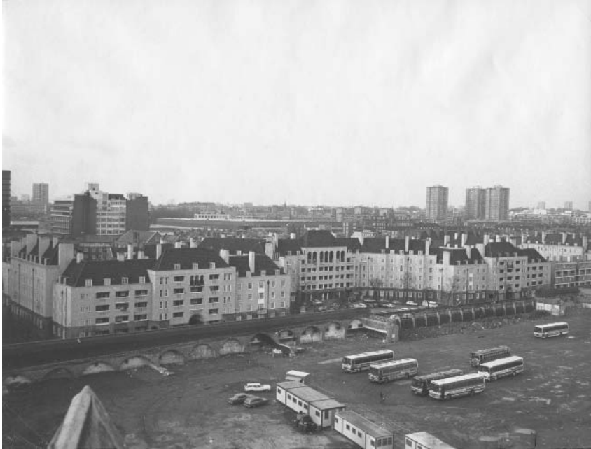
◀ Figure 1.2 View of Ossulston Estate, London, 1927–31
